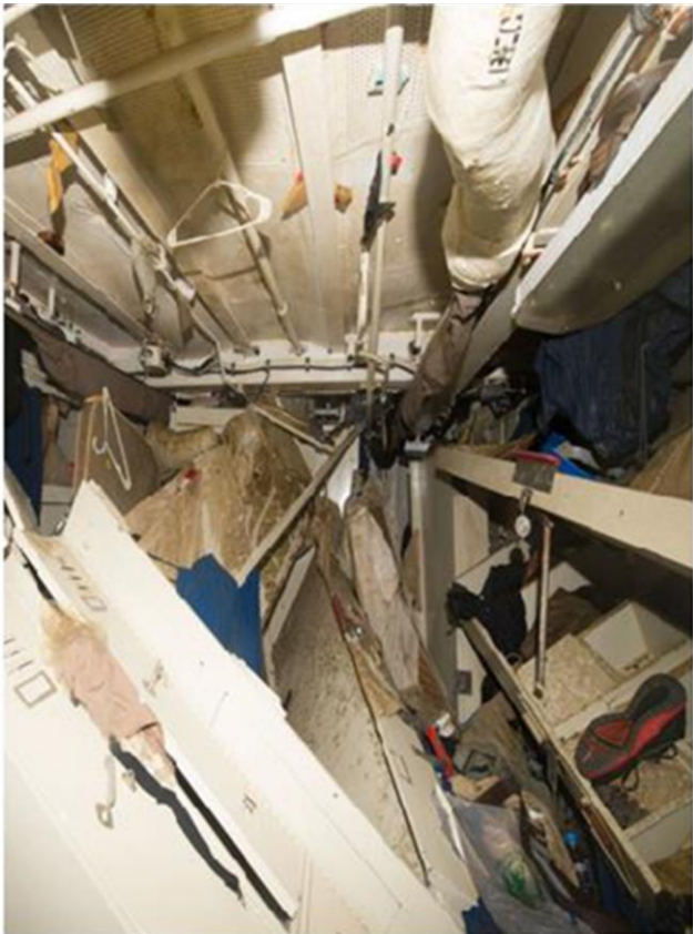
FITZGERALD Berthing 2 Racks Post-Deflooding
