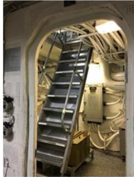
Figure 9 – Non-watertight door frame from Berthing 2 to the ladder going up to Berthing 1 Access Trunk. There is no hatch at the top of this ladder to prevent water from flooding up into Berthing 1.
