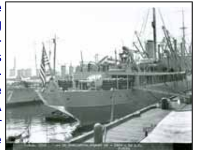
AE-1 at commissioning
